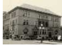
Springfield Chamber of Commerce Building Photograph
